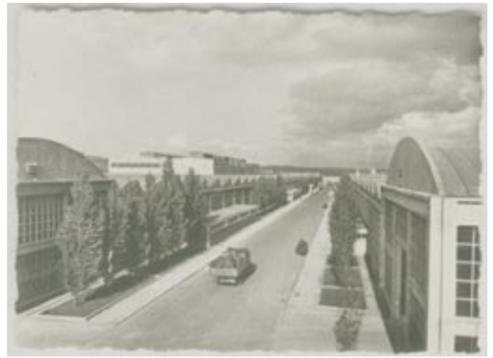
15. (above) Flins. Overall view. This factory was built between 1950 and 1952, and doubled in size in 1955. It employs almost 4000 persons.
