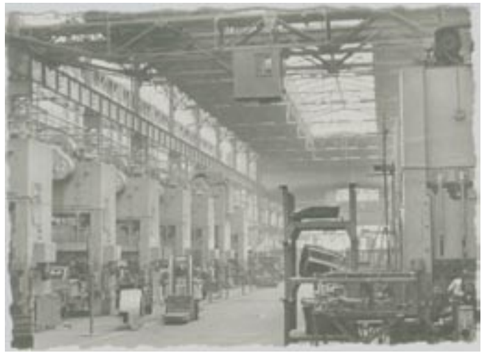
9. Pierre Lefaucheur factory at Flins. Sheet metal presses. The Pierre Lefaucheur plant produces 600 Dauphines daily.
