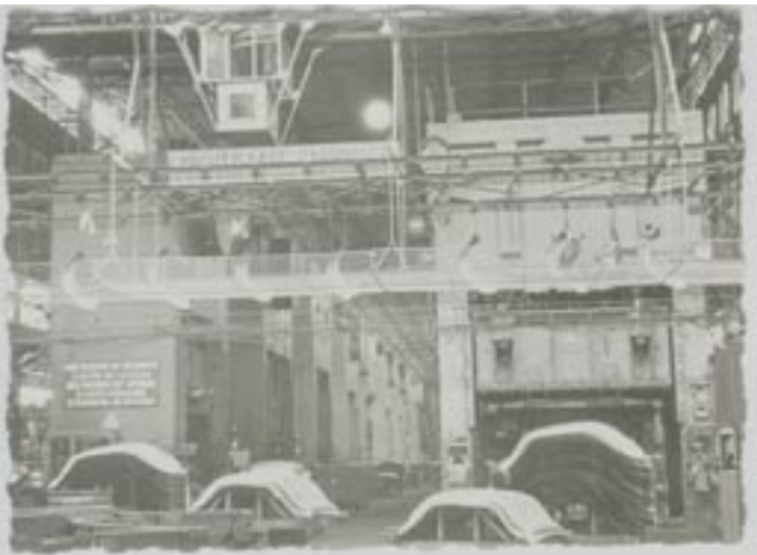
8. (below) Billancourt. Sheet metal presses. Renault consumes 500 metric tonnes of sheet steel daily, 150 tonnes of special steels and 200 tonnes of ordinary steel.
