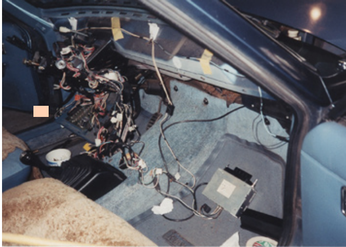
Everything taken out and ready for the A/C installation
